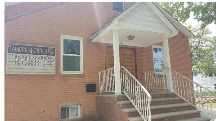
The roof over the front entranceway currently has no gutters. Gutters can be installed and the runoff directed into planter boxes. Additionally, the sidewalk can be converted to pervious pavement. A preliminary soil assessment suggests that more soil testing would be required before determining the soil's suitability for green infrastructure.
