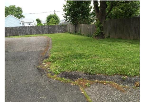
Parking spaces can be replaced with pervious pavement to capture and infiltrate stormwater. Downspouts in the front of the smaller building can be directed into a rain garden to capture, treat, and infiltrate runoff. A preliminary soil assessment suggests that the soils have suitable drainage characteristics for green infrastructure.
