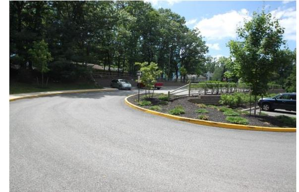
The parking lot is new but can be converted into pervious pavement in the future. A rain garden can also capture, treat, and infiltrate runoff, and downspouts can be disconnected onto existing landscaping. A preliminary soil assessment suggests that the soils have suitable drainage characteristics for green infrastructure.
