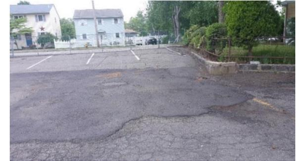
A small garden behind the church is currently being watered by a disconnected downspout. This area could be turned into a larger rain garden. The parking lot is in fair condition and can be converted into pervious pavement. A preliminary soil assessment suggests that the soils have suitable drainage characteristics for green infrastructure.
